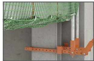
Double post construction at end post.
