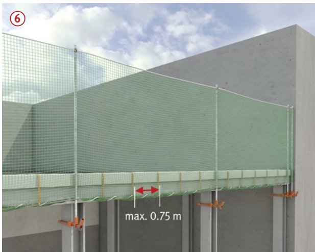
Edge protection fastened to components at bottom.
